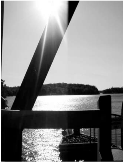
Wasuaksing First Nation Swing Bridge – June 2010 (photo)
